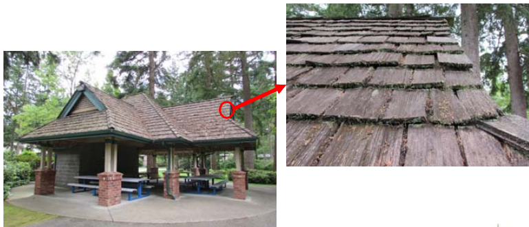
Existing Cedar Shake Roof
